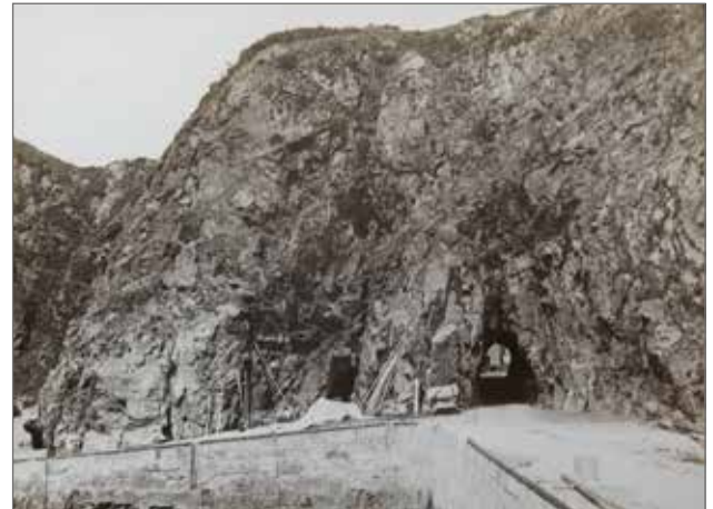
The Tunnel, Creux Harbour 856A0762.jpg Donated by Deryck Hamon, 2024
