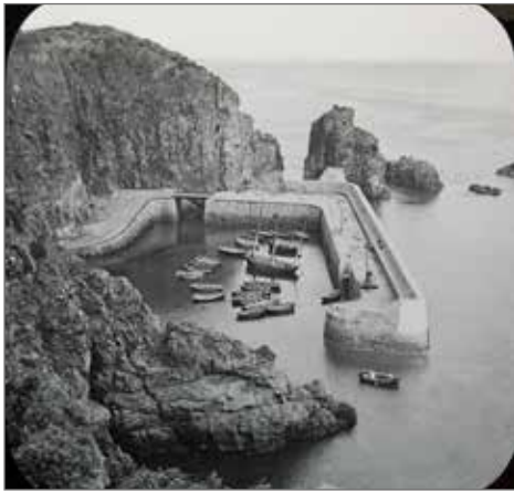
Creux Harbour, Sark (Harbour was completed c 1870, bridge filled in, sally port & second pierhead added in 1893. 4 copies) 856A0771.jpg (& 72, 74, 75) Donated by Deryck Hamon, 2024
