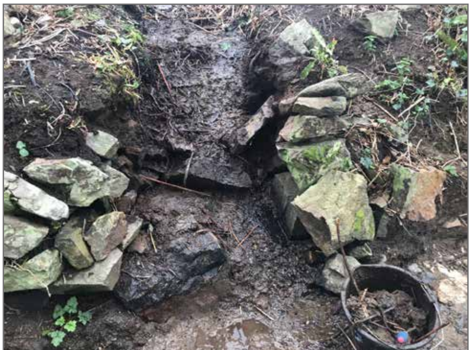
Clearing the channel into the lavoir
